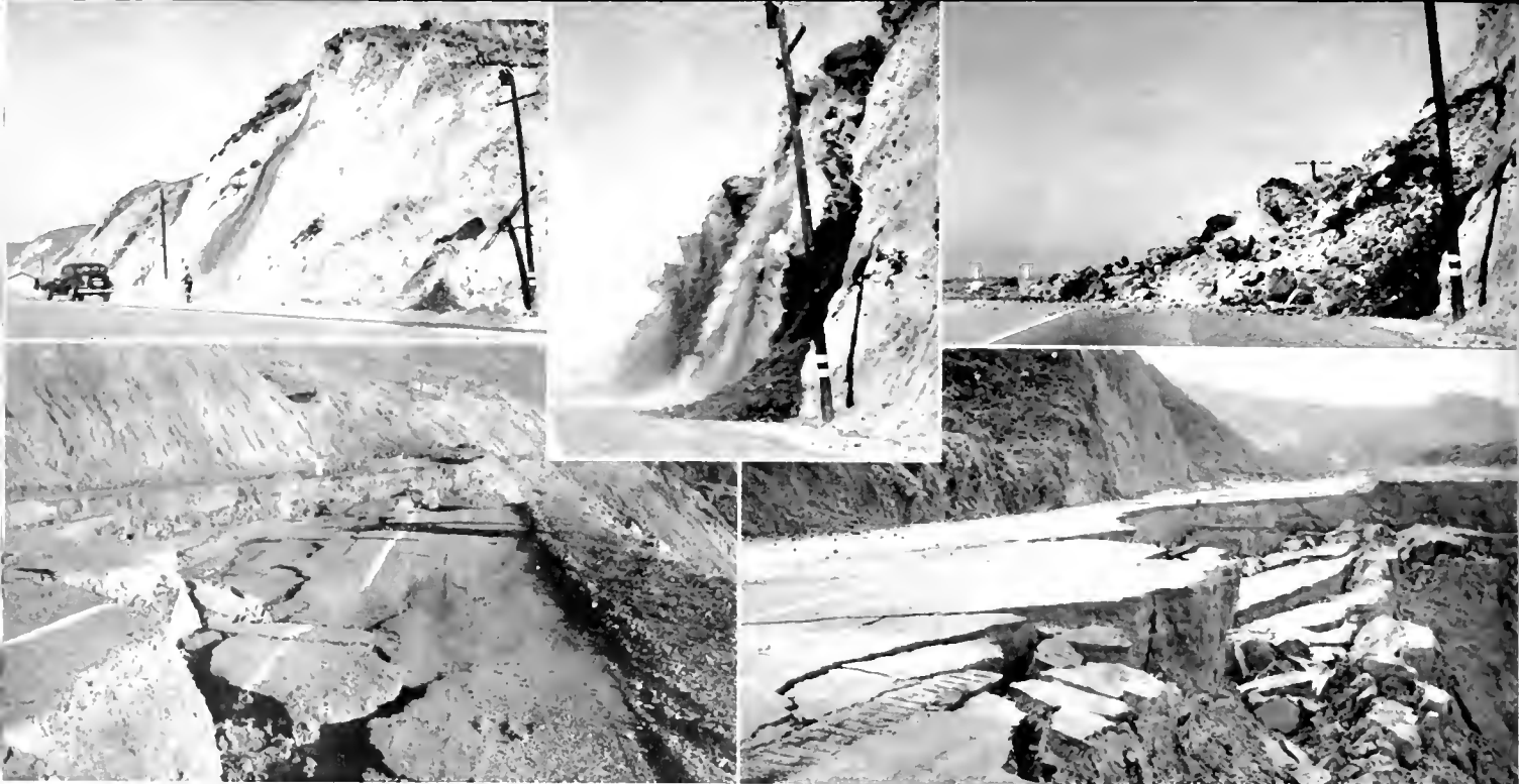
The upper three pictures show a slide in progress south of Topanga in Los Angeles County. Lower pictures show hazard and extent of typical slipouts. Sketch shows method of correction
